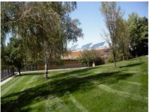
The Energy & Sustainability Office is currently working on two solar projects. The Swenson Gym solar thermal project (pictured above) will use solar panels to heat the pool. The panels will produce roughly 1,000 decatherms of energy annually which equates to saving the University about \$7,000 - \$10,000 a year in heating costs.
